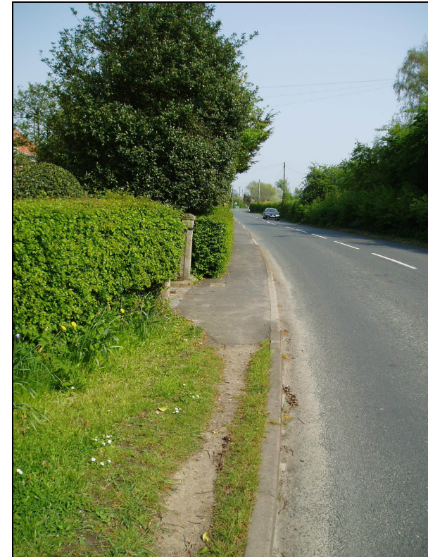
Figure 4 : Start of footway outside No. 107 Temple Lane
